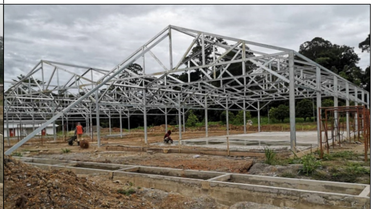
Concreting the floor of the greenhouse
