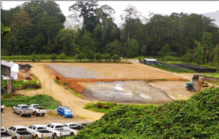
Site preparation for greenhouse construction.
